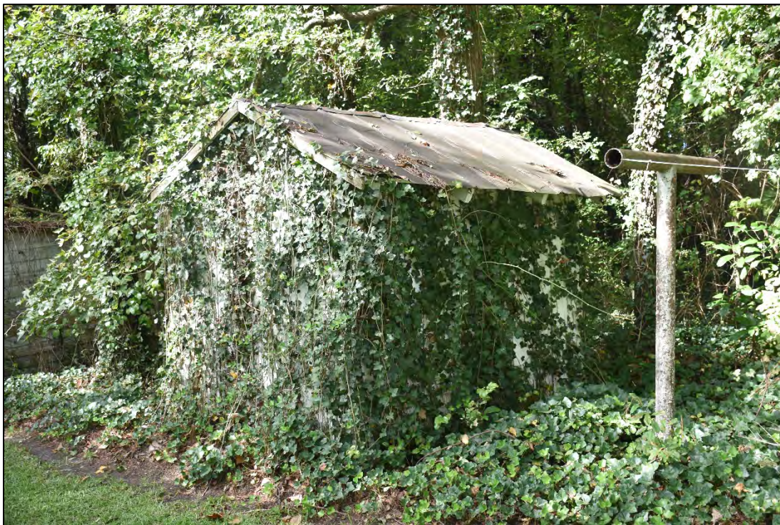
Figure 2.1.60. Jack Douglas House (BF1412), shed, facing southeast.
