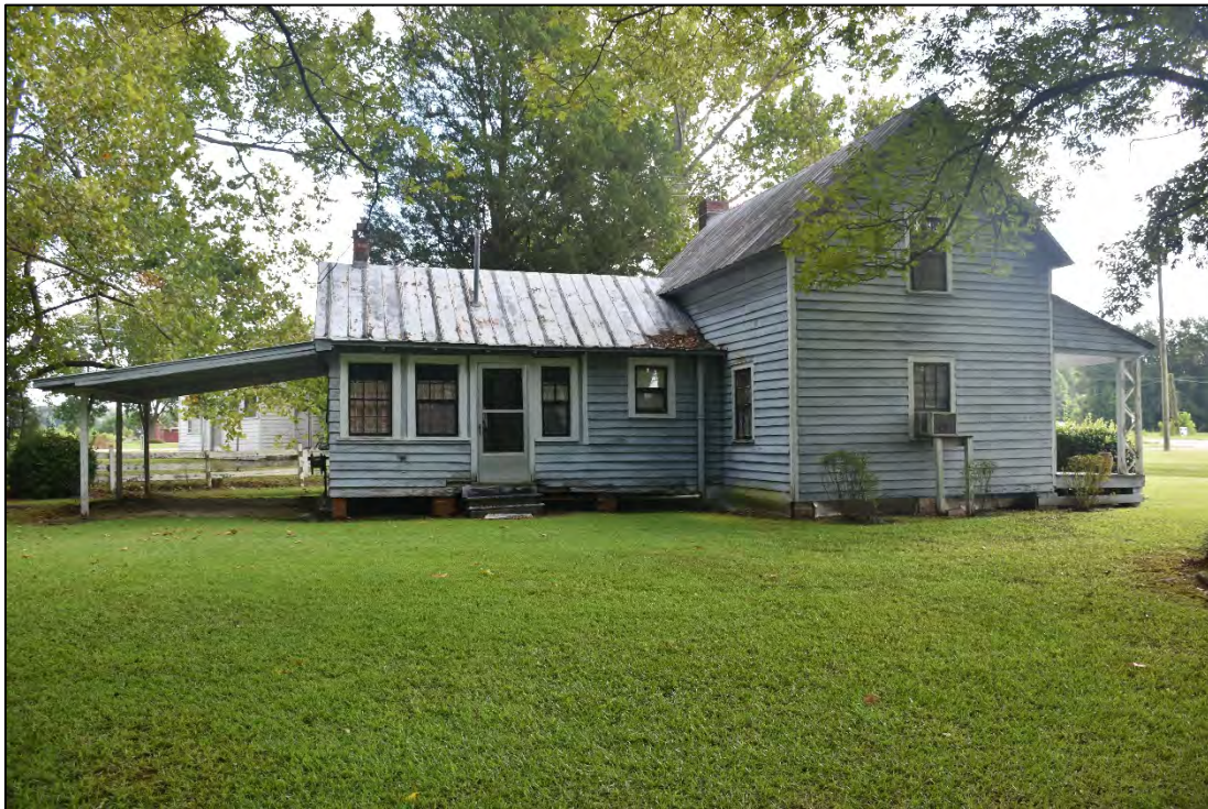
Figure 2.1.53. Jack Douglas House (BF1412), facing north.
