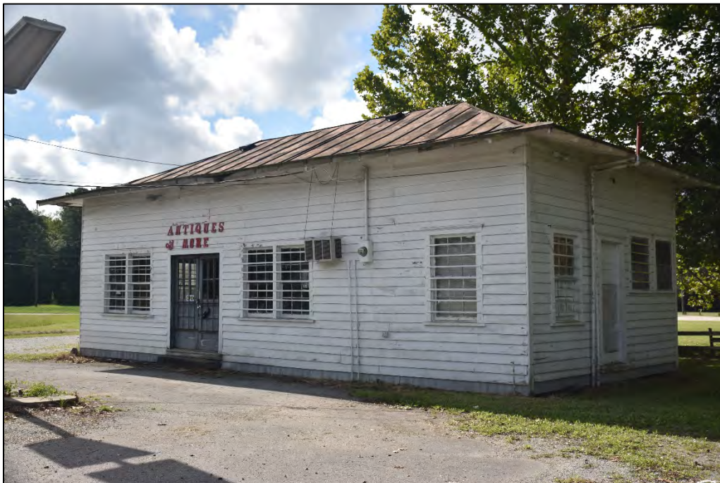
Figure 2.1.37. Douglas Crossroads Store (BF1404), facing southeast.
