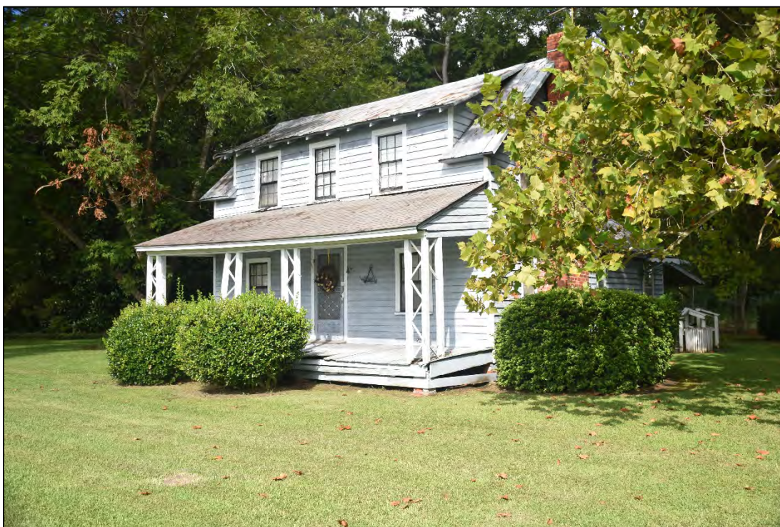
Figure 2.1.57. Jack Douglas House (BF1412), facing southwest.
