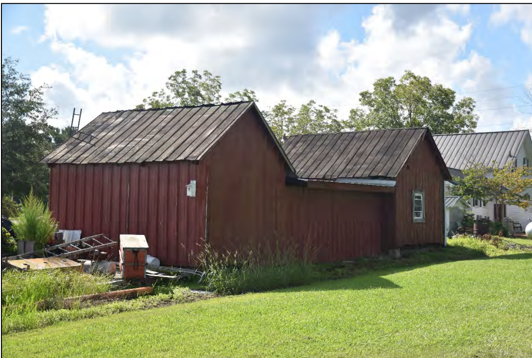
Figure 2.1.18. Douglas Farm (BF1400), circa-1920 shed and well house, facing southeast.
