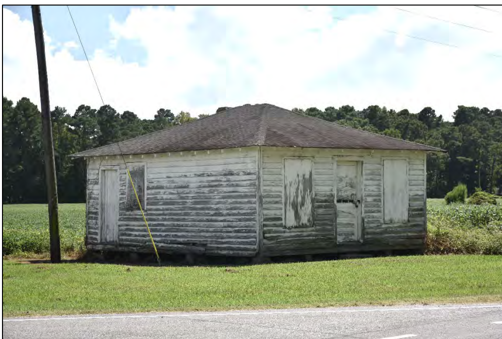
Figure 2.1.43. Store (BF1317), intersection of NC 99 and Rest Haven Road, facing south.
