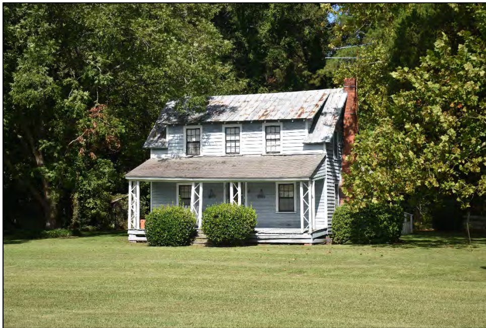
Figure 2.1.29. Jack Douglas House (BF1412), facing southwest.
