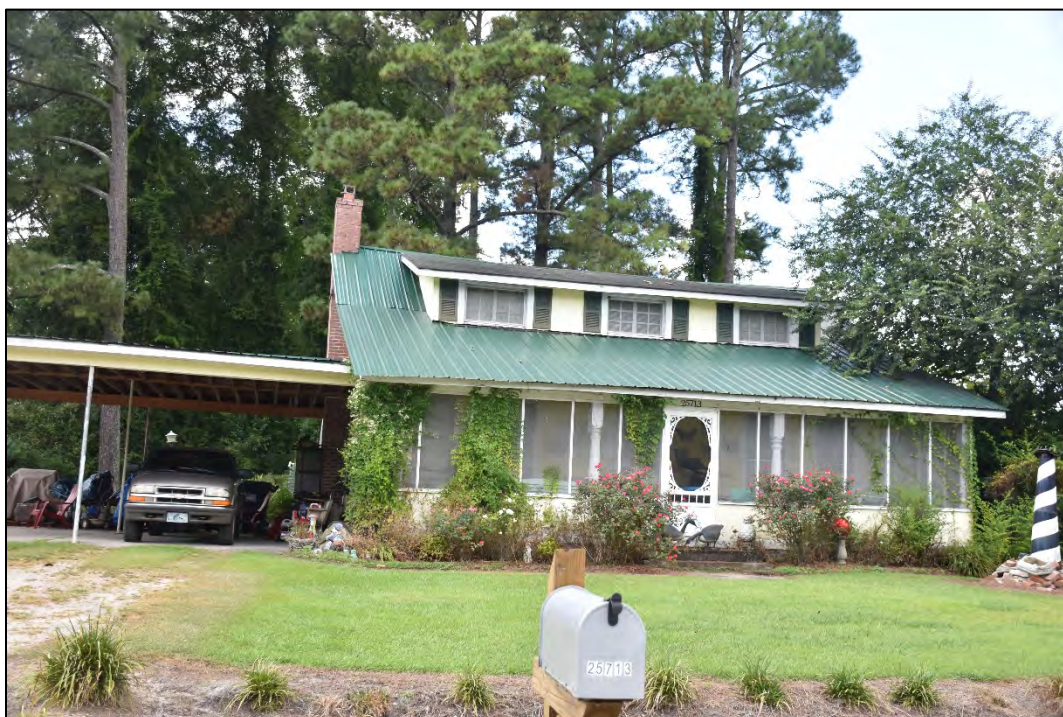
Figure 2.1.64. House at 25713 US 264, Pantego (NSN), facing west.
