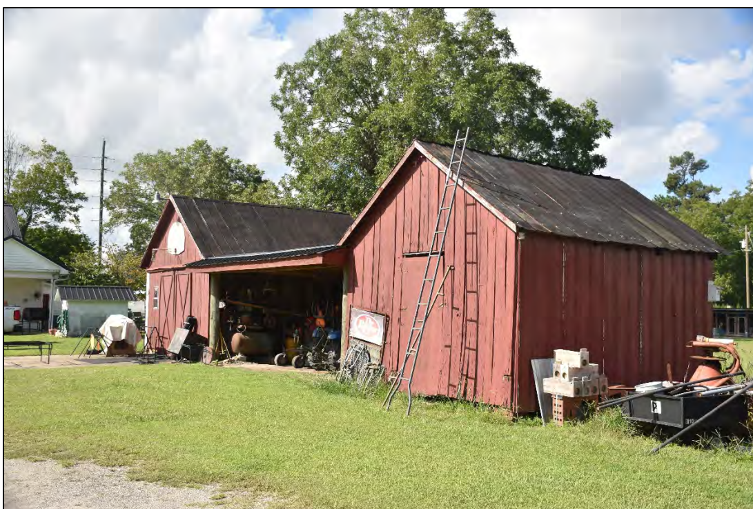
Figure 2.1.20. Douglas Farm (BF1400), circa-1920 shed, facing southeast.
