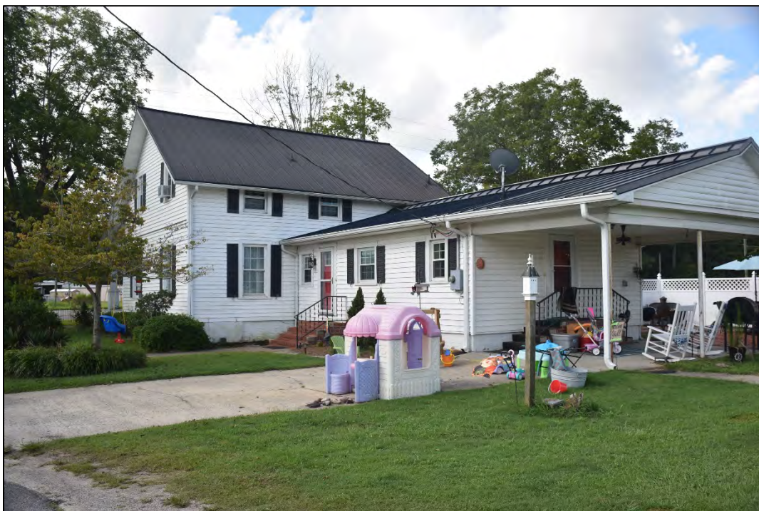
Figure 2.1.14. Douglas Farm (BF1400), house, facing southwest.
