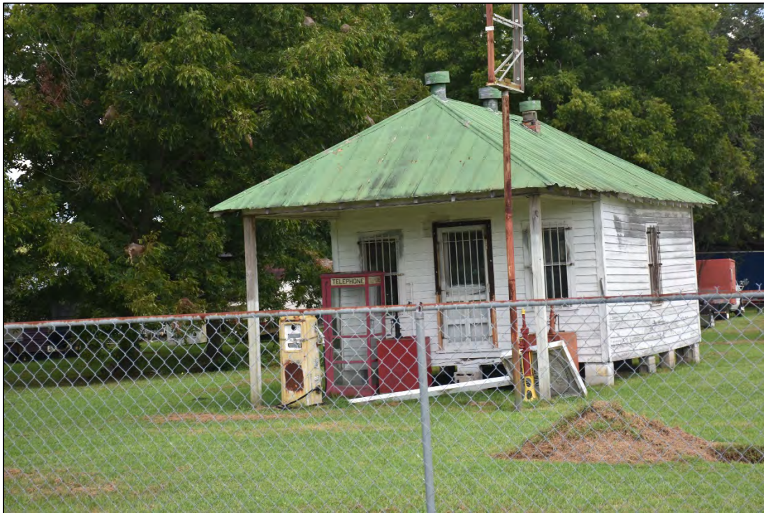
Figure 2.2.44. Joe Toler Store (BF1645), facing north.
