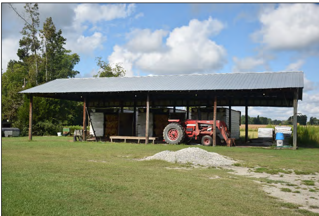
Figure 2.1.21. Douglas Farm (BF1400), tobacco shed and bulk storage, facing west.
