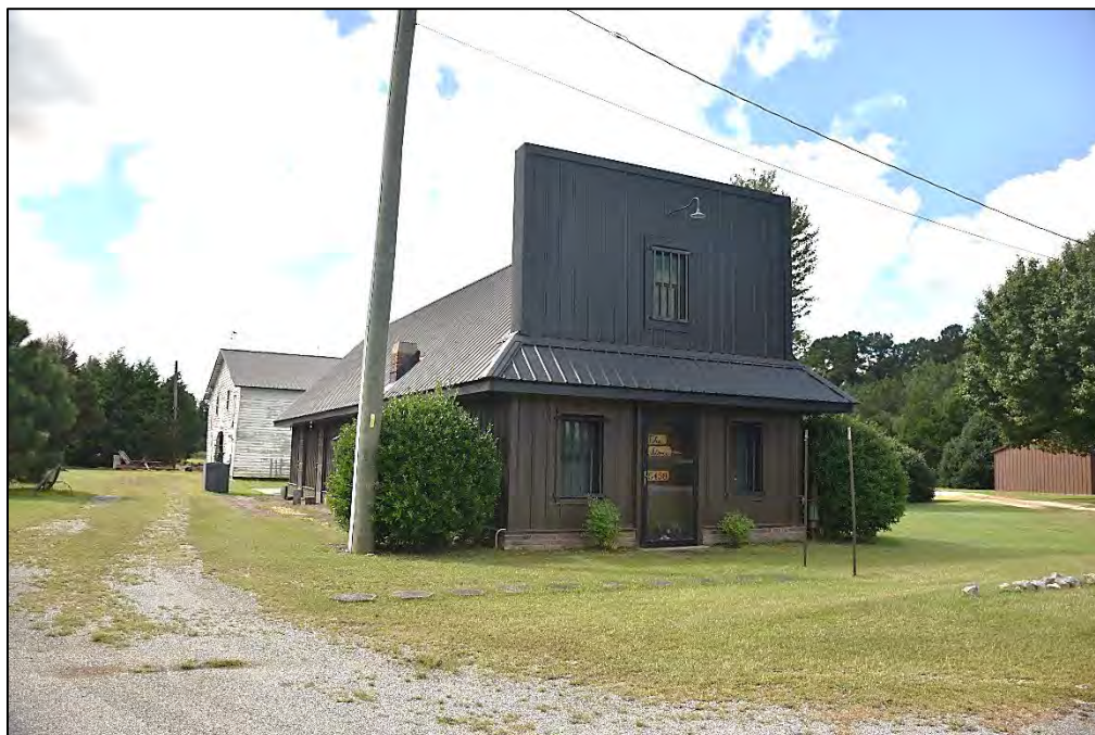
Figure 2.2.45. Store (BF1325), south of Slatestone Road, facing southwest.
