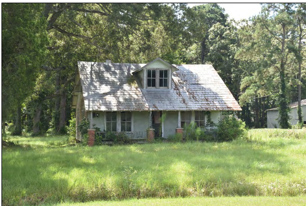
Figure 2.1.65. House (BF1378), facing south.
