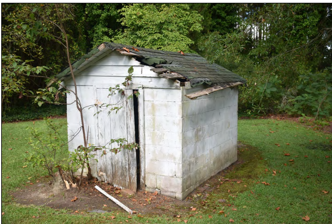
Figure 2.1.58. Jack Douglas House (BF1412), well house, facing southwest.
