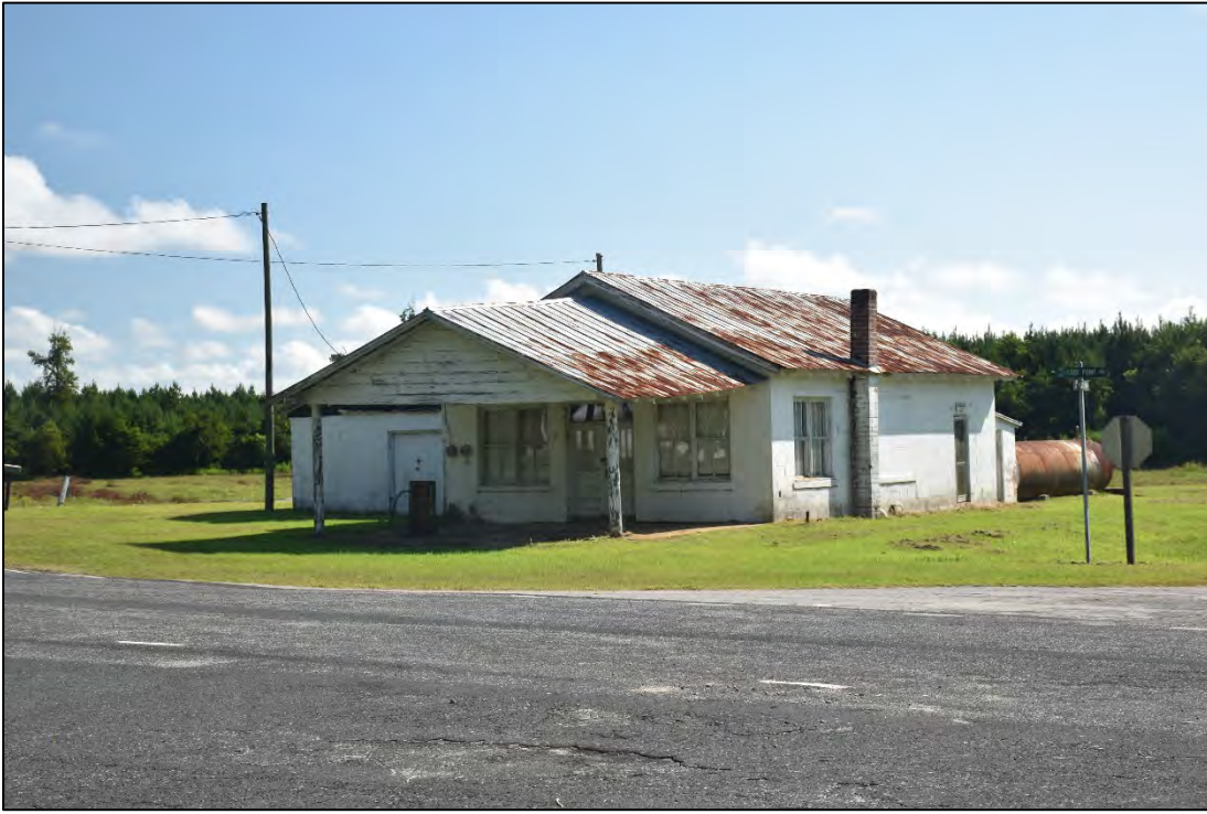
Figure 2.2.48. Pipkin Store (BF1755), facing east.
