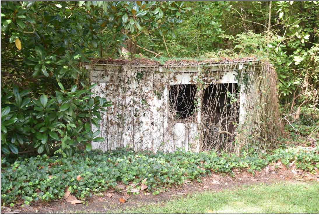
Figure 2.1.61. Jack Douglas House (BF1412), chicken coop, facing south.
