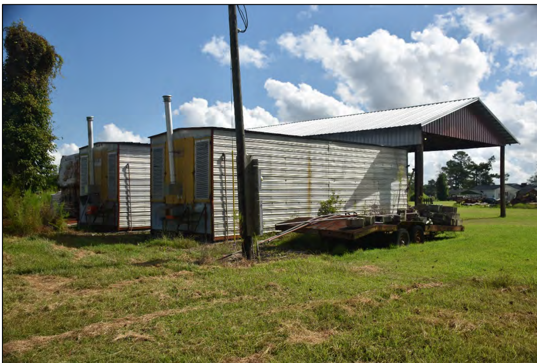
Figure 2.1.22. Douglas Farm (BF1400), tobacco shed and bulk storage, facing northeast.
