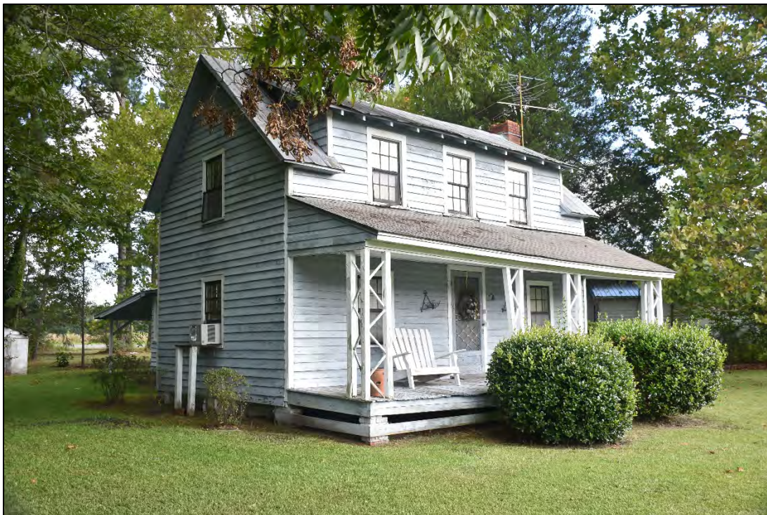
Figure 2.1.52. Jack Douglas House (BF1412), facing northwest.
