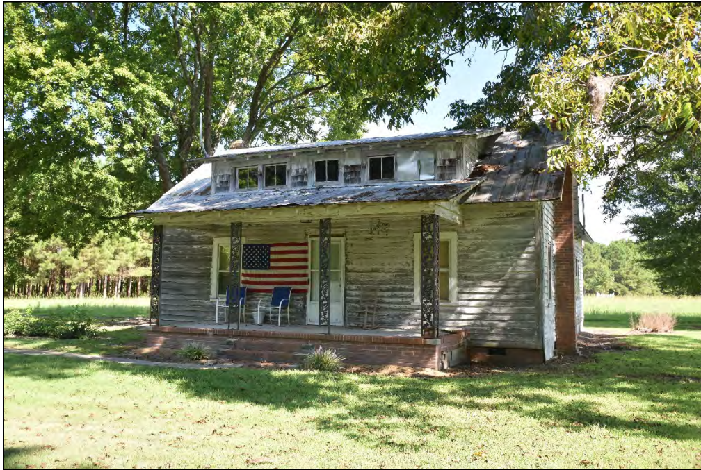
Figure 2.1.68. Brame-Boyd House (BF1691), facing northwest.
