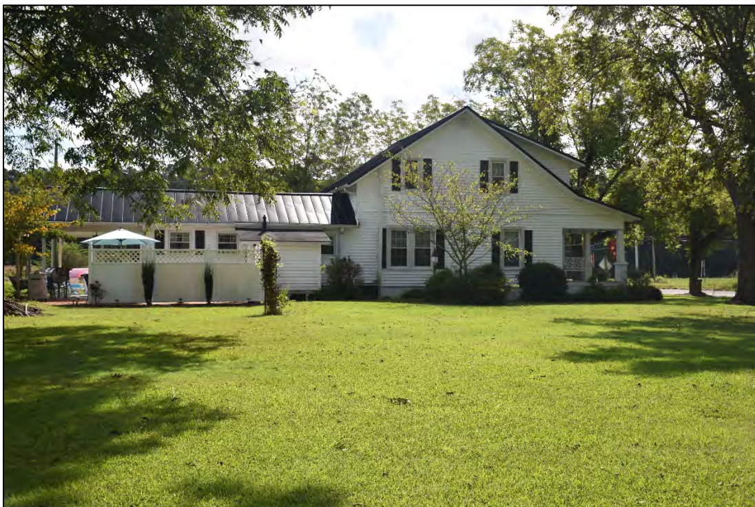
Figure 2.1.15. Douglas Farm (BF1400), house, facing east.
