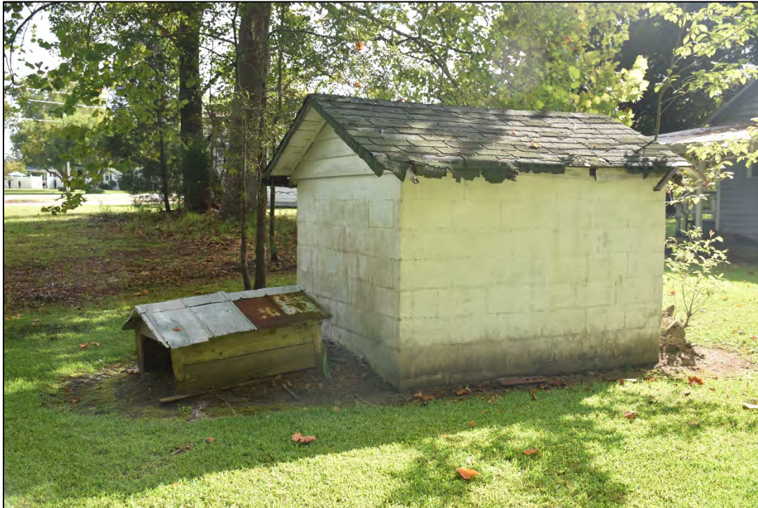
Figure 2.1.59. Jack Douglas House (BF1412), well house, facing northeast.
